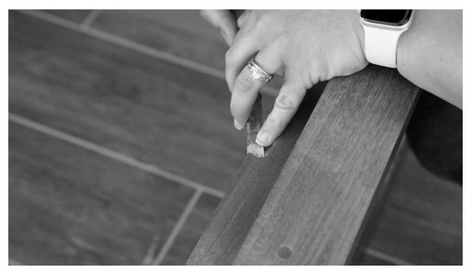
When the bed is lowered, the wing nuts holding the handles in place may hit the cleat at the foot of the bed. To remedy this, use a 1/2" forstner drill bit to drill holes approximately 1/4" deep, overlapping each other. This creates a notch for the wing nuts to fit and the bed frame to sit flush on the cleats. Clean up the notches with a chisel.
