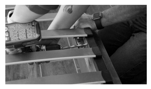
Set the bed frame onto the lift mechanism, with the angle braces to the inside edge of the bed frame sides. Using the pre-punched hole sin the braces as a guide, drill three 25/65" holes through the bed frame in three places on each side of the bed (one on each end and one in the middle). Attach the bed frame to the punched angle brace using the six included bolts, washers, and nuts in the hardware package.
