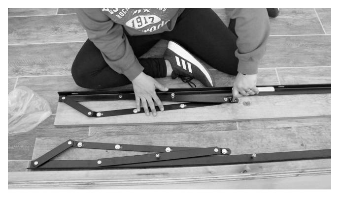
Attach the lift mechanism to the cleats using 3/4" long by 5/16" bolts and washers.
